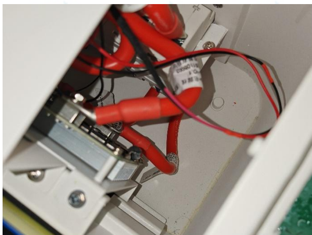
No.6.5-3 Inspection after test (No water ingress)
