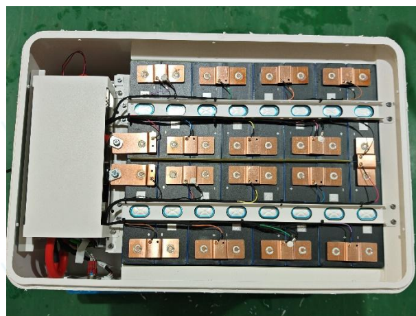
No.6.5-2 Inspection after test (Upper cavity)
